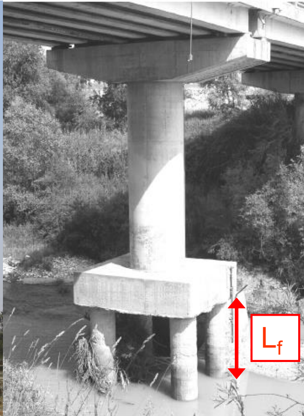
RIVER FOUNDATION, SCOUR ( L_f = \text{Limited} )
